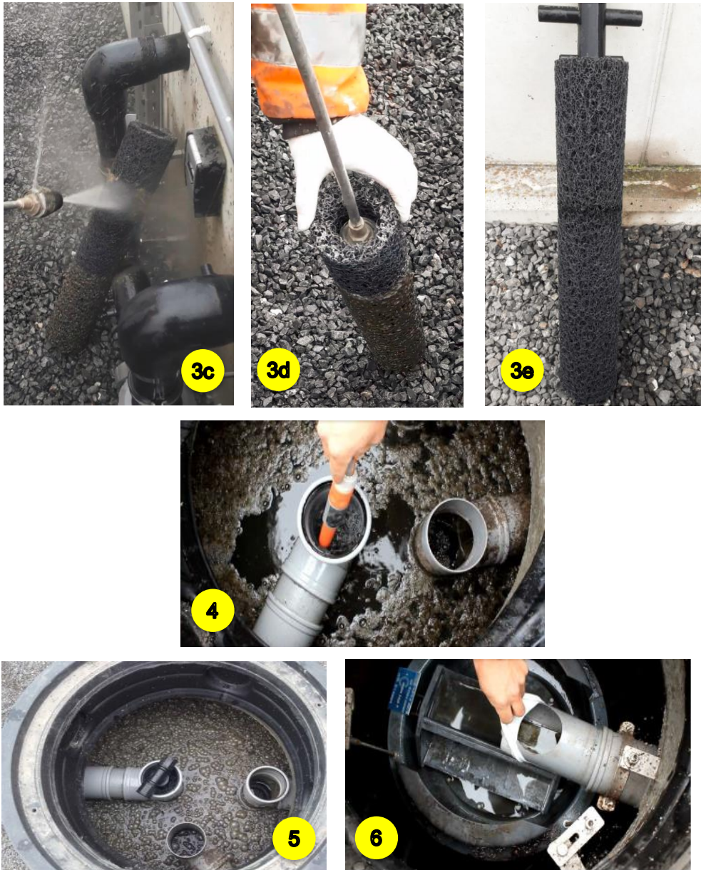
Fig-14 : Cleaning steps of the effluent filters
