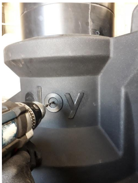
Fig.15 – percement de la rehausse
